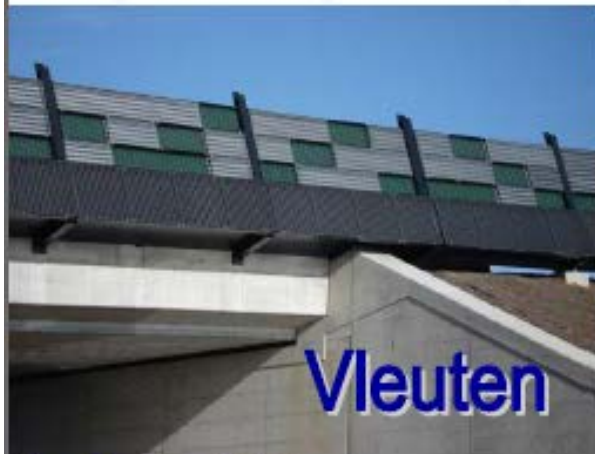
Sound absorbing noise barrier
